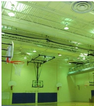
The school's LED retrofit proved to be a simple and rewarding process. Each HPS high bay and ballast was replaced by an RVLT LED high bay, which vastly improved the gym's lighting quality. Under the old HPS high bays, footcandle readings in the 24-foot-high gym ranged from 9.8 to 25.5.
