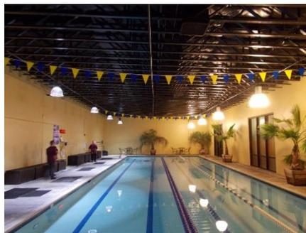
The previous inefficient lighting consisted of high bays and tube lights used for general illumination in the interior of Meniffee Valley Athletic Club. The exterior parking lot also needed more efficient street lighting. The older conventional fixtures were replaced with 44 RVLT LED lighting products. RVLT 15-watt LED tube lights and 100-
