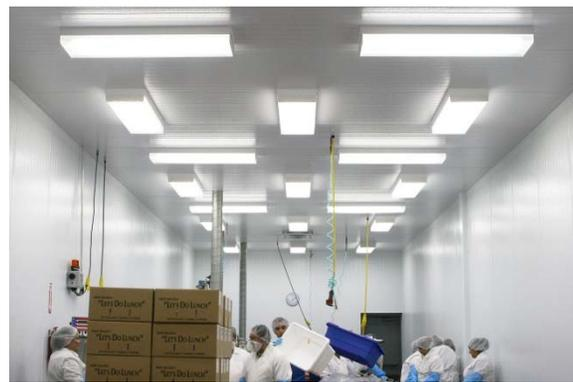
RVLT's LED lamps have enabled IFS to surpass the USDA-required 100 footcandles of illumination. Under the RVLT T8s, light levels actually reach 105 footcandles.
